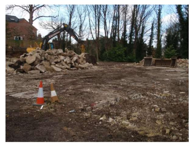
Plate 4. The site showing concrete slabs being broken up
